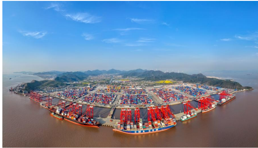
The Dapukou Container Terminal in Jintang port area has been completed as a fully automated terminal featuring port-wide mixed-line operations 金塘港区大浦口集装箱码头建成全域混线作业自动化码头
