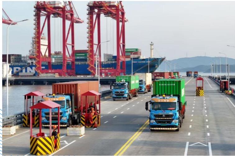
Meishan Port Area has completed construction of a single-body, multi-million TEU-capacity automated container terminal capable of mixed-line operations 梅山港区建成单体超千万混线作业自动化集装箱码头
